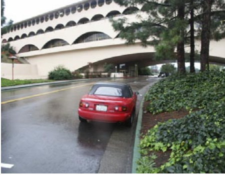
Sightline to Building Entry
