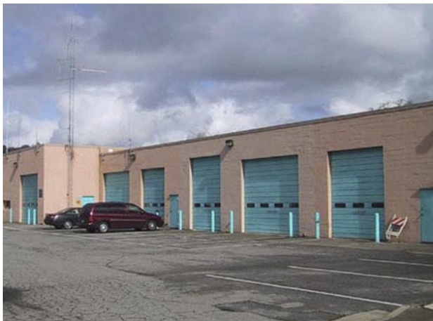
1. County General Services Building
