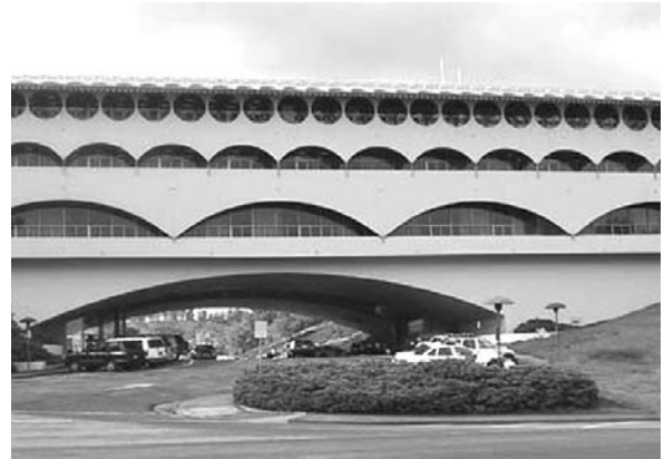
Hall of Justice Entry Arch - 1970
