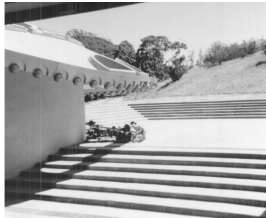
South End of the Administration Building - 1970
