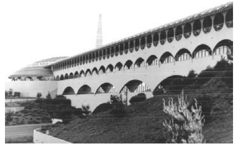
View of Administration Building
