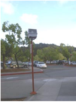
Non-historic parking lot light fixture with additional pole mounted floodlight for security lighting purposes at county jail facility
